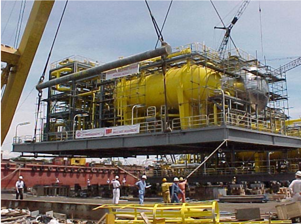
Figure 7 - Deflection Topsides Module in 4-point-lift
