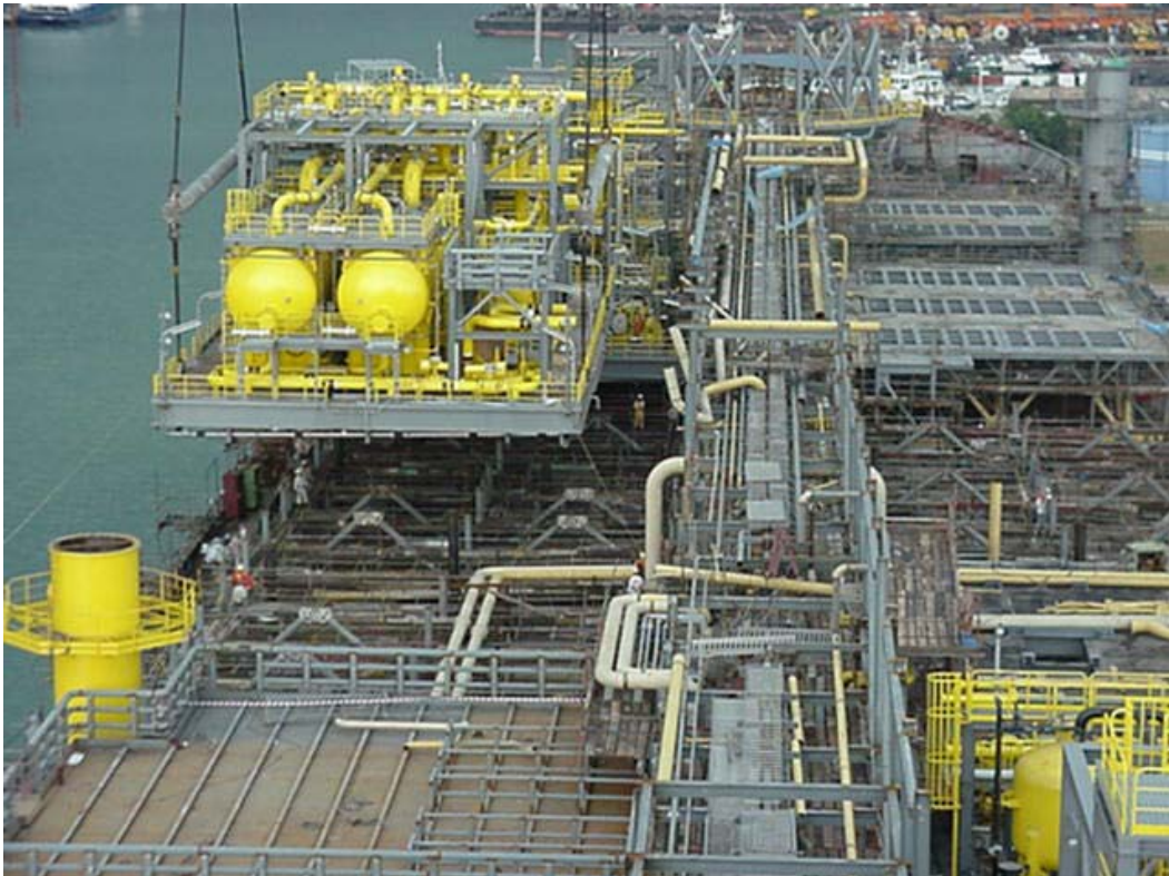
Figure 8 - Module Installation on Column Support
