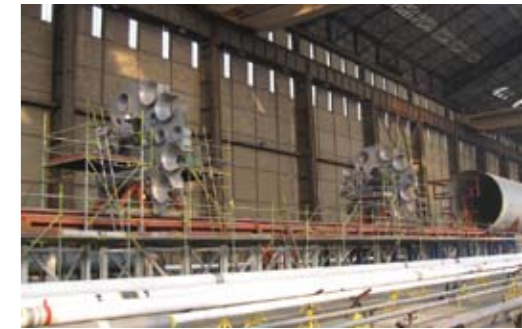
Construction of caisson
