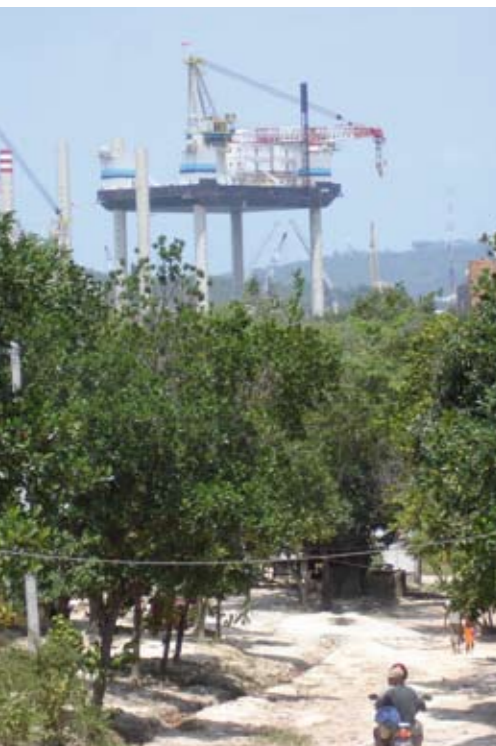
Full height test JB-110 at Labroy Shipyard in Batam
