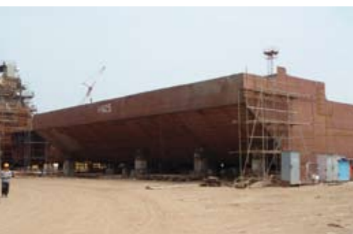
Building of the JB-115
